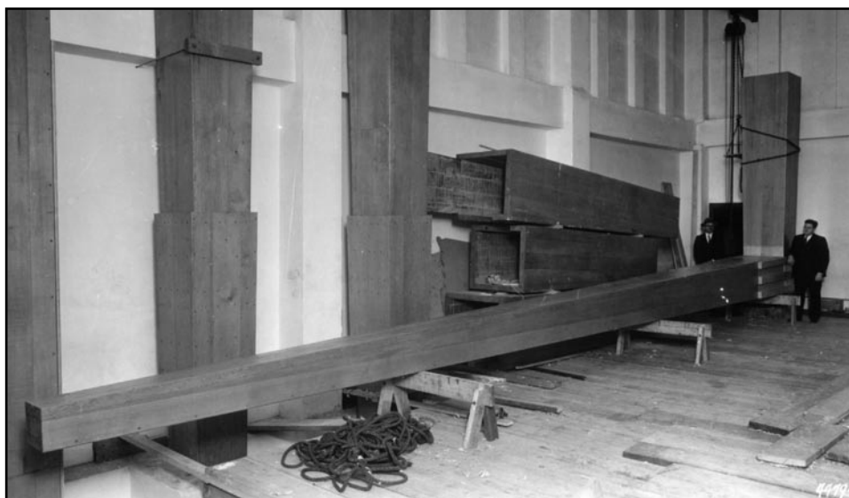
This pipe – part of the 64-foot rank – is thought to be the GGGGG note (42-2/3)
