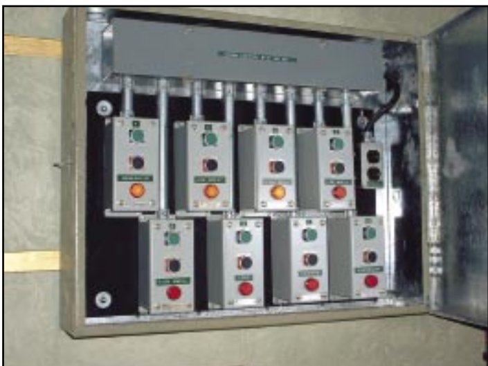
Starter switches for the organ. They control 600 horsepower for the blowers and 5 horsepower for the DC generator. Hang on to your hats!
