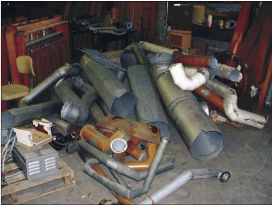
Windlines that were cut out of the organ during the renovation. These windlines were partially for the left relay as well as the left Gallery chambers. New routings for these windlines will have to be established.
