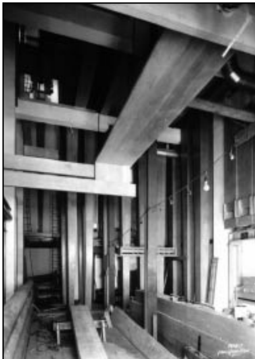
At floor level in the Right Stage chamber. Gradually, more and more of the 64-foot stop's pipes are built and maneuvered into position, but they are still without their boots. On the right (aligned with the light bulb) is the CCCCC# pipe, with CCCCC next to it. Arrayed across the picture (left to right) are the pipes for notes GGGGG# down to DDDDD (the latter being positioned next to CCCCC).
