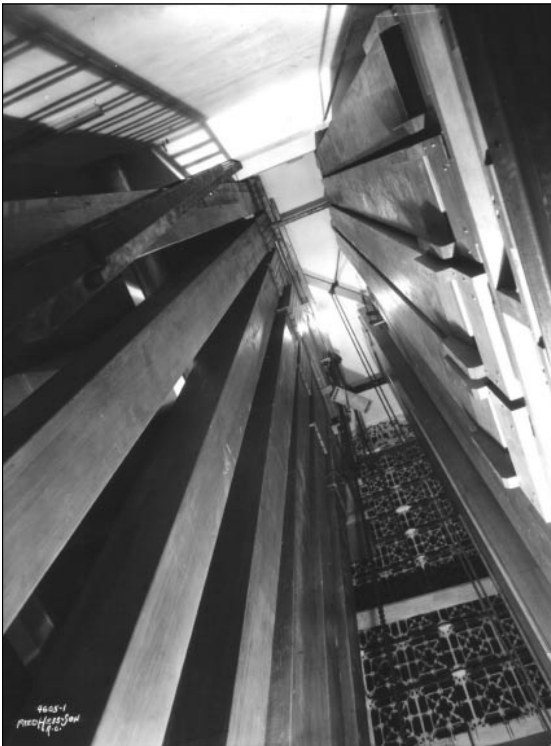
Looking up at the DDDDD to GGGGG# pipes. These pipes range in length from 56\frac{8}{9}' to 40\frac{24}{25}' . Due to the camera angle, the pipes look straight but, actually, they are flared. On the right are pipes belonging to the 32-foot octave of the Great organ's Sub Principal .
